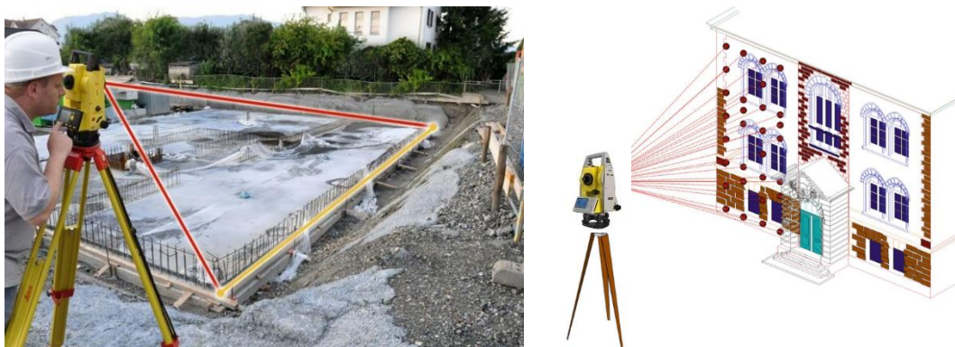
Figure 4. Staking out with tachymeter and As-built survey
